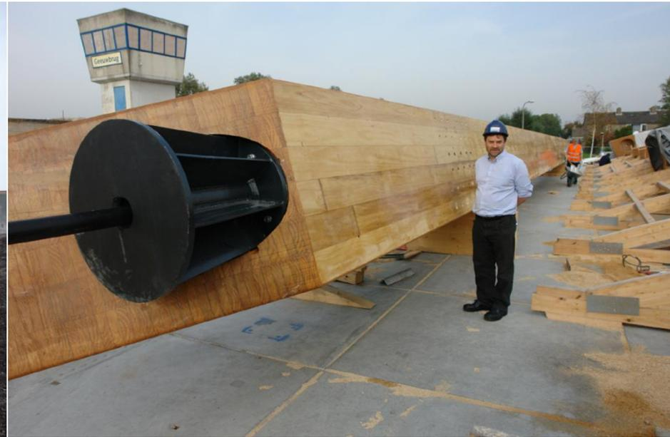
Sneek bridge – element. The bridge is made from Accoya – modified wood
